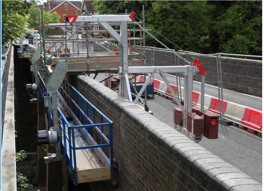
A bespoke suspended access solution from Harsco Infrastructure is helping keep both road traffic on the bridge and rail traffic below the bridge on the move during a major bridge repair project in Hampshire. Harsco has designed and built a system which uses twin cradles suspended over the sides of the Church Lane East railway bridge in Aldershot. This provides safe and flexible access for refurbishment work.
